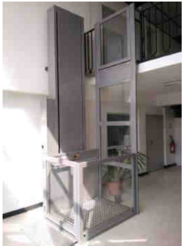
Wall fixing of the drive tower for a space saving installation
